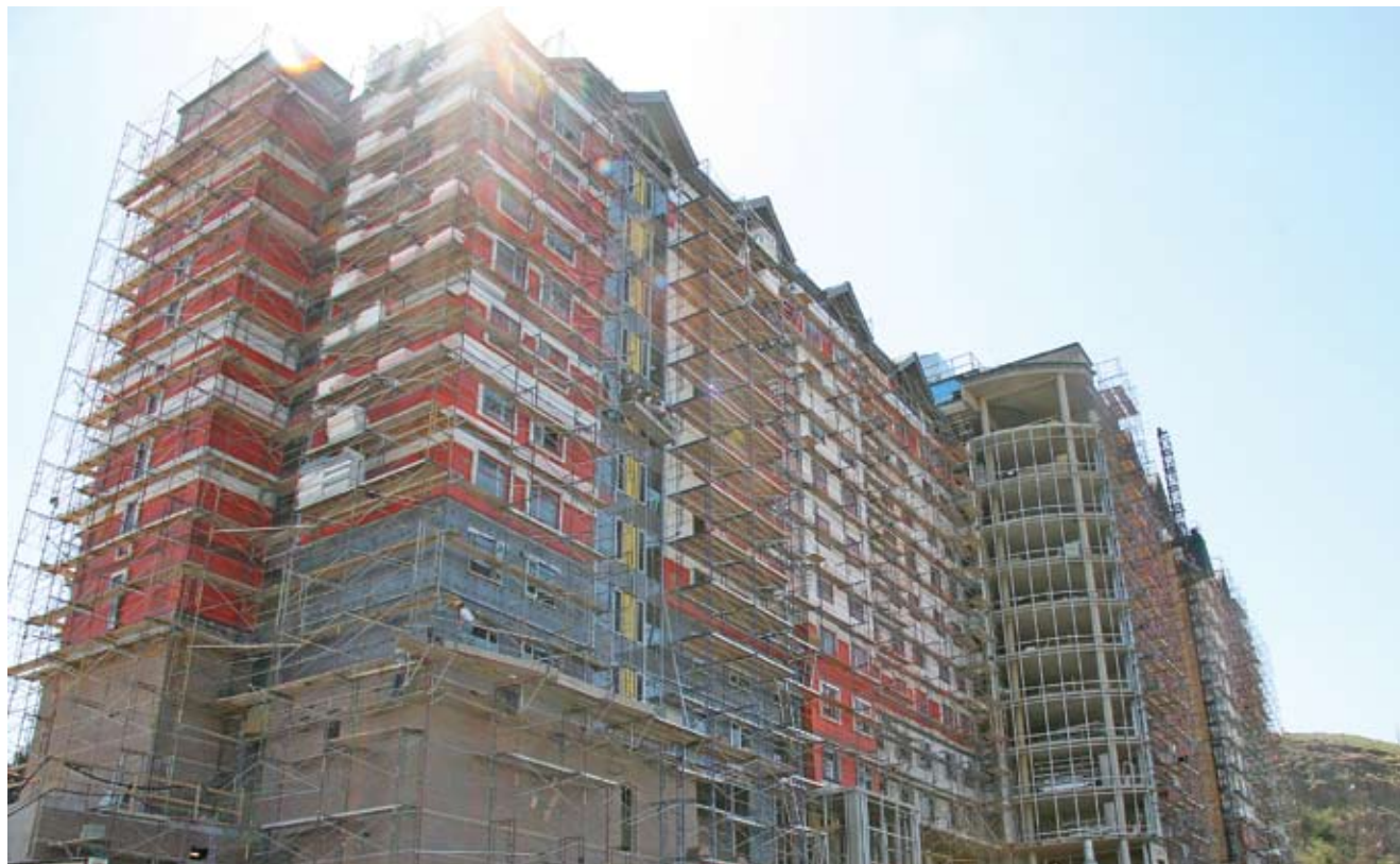
New residence for domestic and international students
